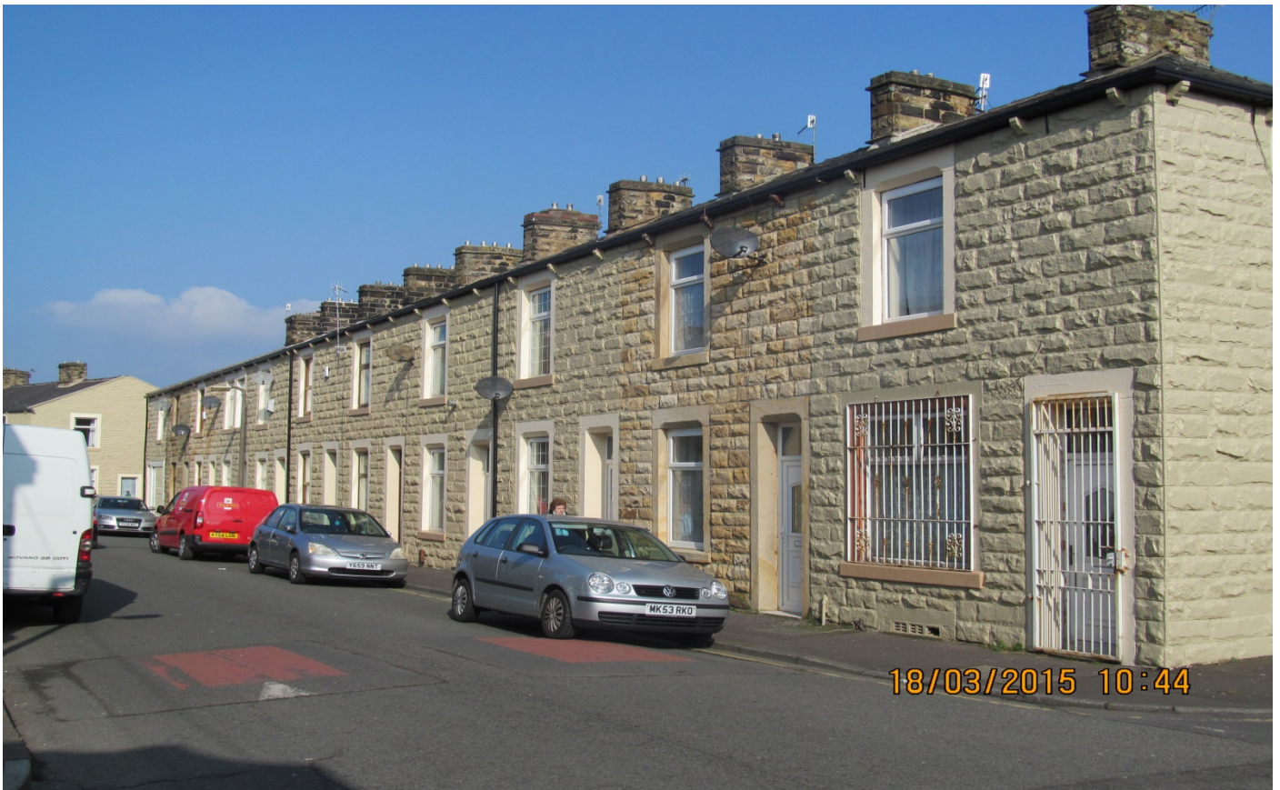
Photograph 2 Upon completion of the Brennand Street painting scheme.
