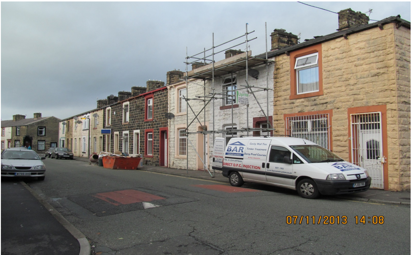
Photograph 1 Prior to the Brennand Street painting scheme.
